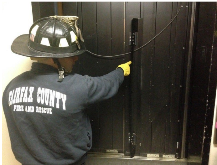
Figure 7. Elevator door vane.
