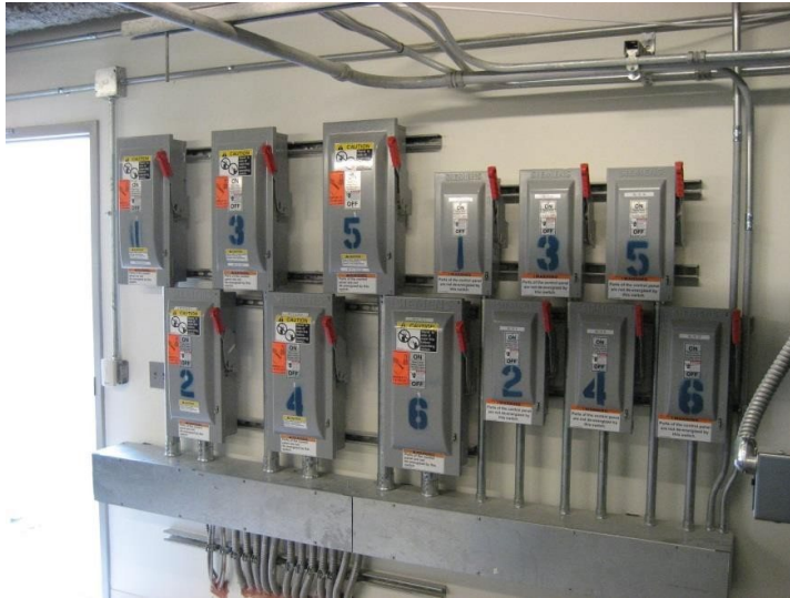
Figure 12. Mainline disconnect.
