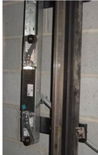
Figure 8. Final limit switch.
