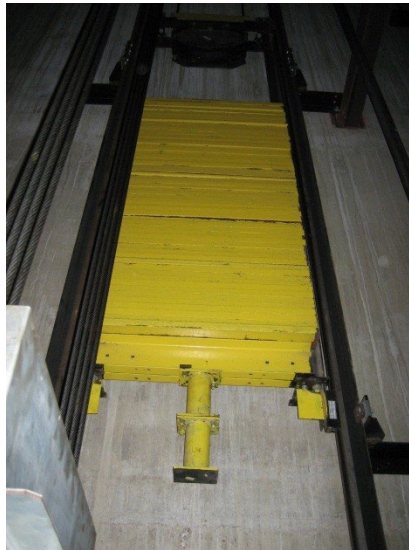
Figure 5. Example of a counterweight.
