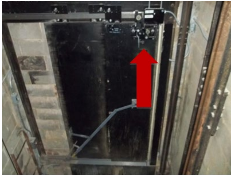
Figure 11. Interlock device.
