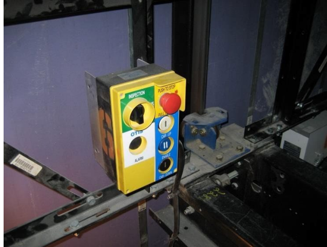
Figure 10. An example of an inspection station.
