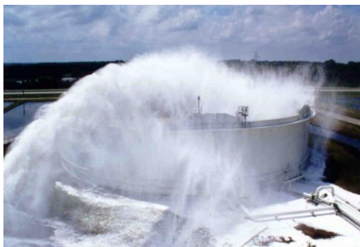
Figure 19: Type III foam application.
