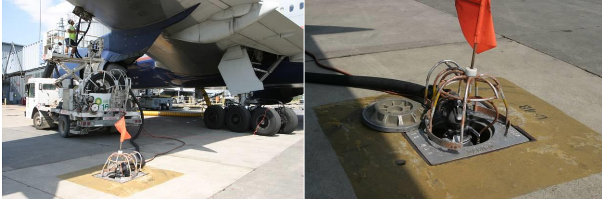
Figure 10: Examples of airport fuel hydrants.
