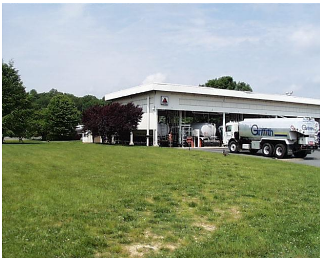
Figure 2: Tanker truck at loading facility.
