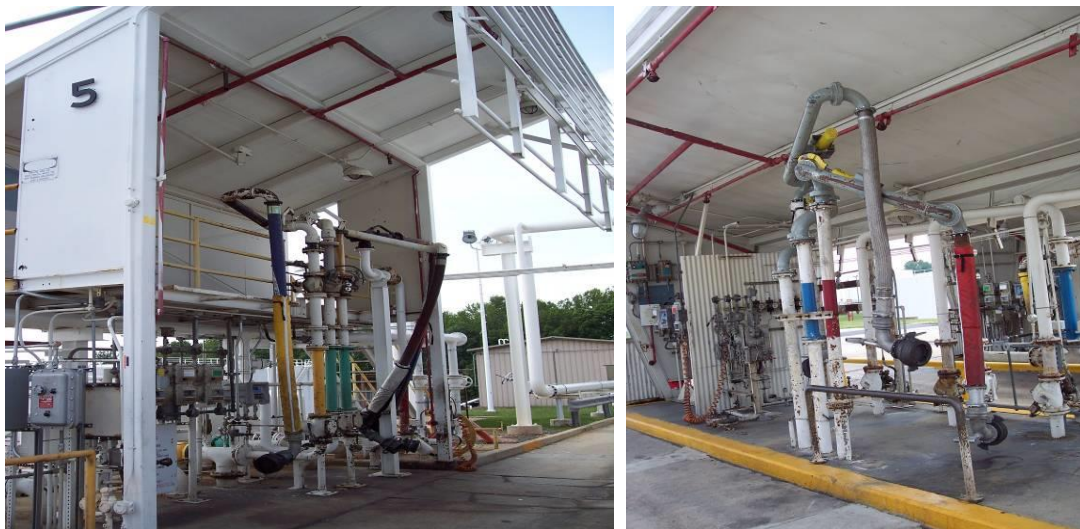
Figure 11: Typical loading racks found in the NOVA region.
