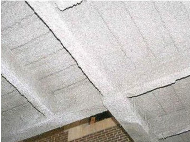
Figure 12. Spray-on fireproofing.
