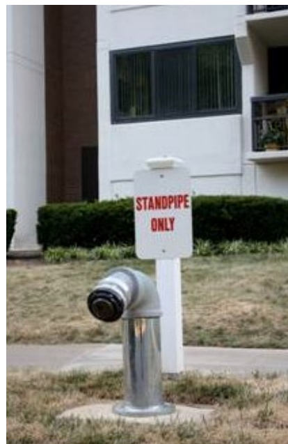
Figure 23. Large-diameter hose connection.
