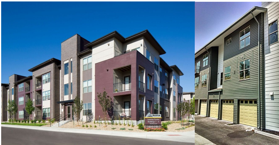
Figure 46. Side Alpha (left) and side Charlie (right) of a walk-up midrise building.
