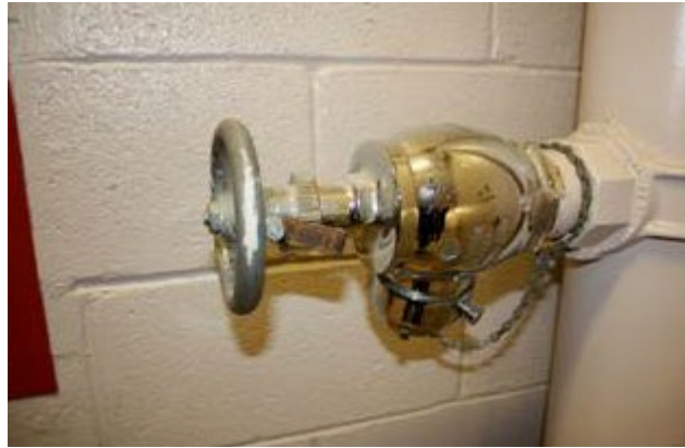
Figure 28. Pressure-reducing valve.
