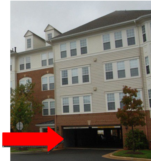
Figure 51. Parking garage access.
