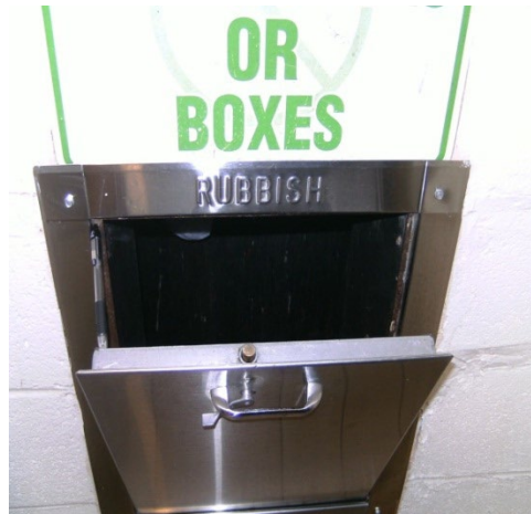
Figure 35. Trash chute.
