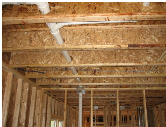
Figure 42: Plywood I-beams, Commonly Called “Ply-Is”
