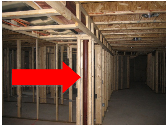
Figure 41: This Metal Column Supports the Overhead Girder
