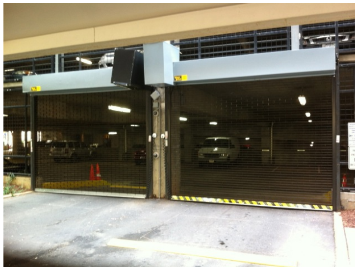
Figure 66: Mid-rise Parking Garage Secured with Large, Metal, Automatic Gate
