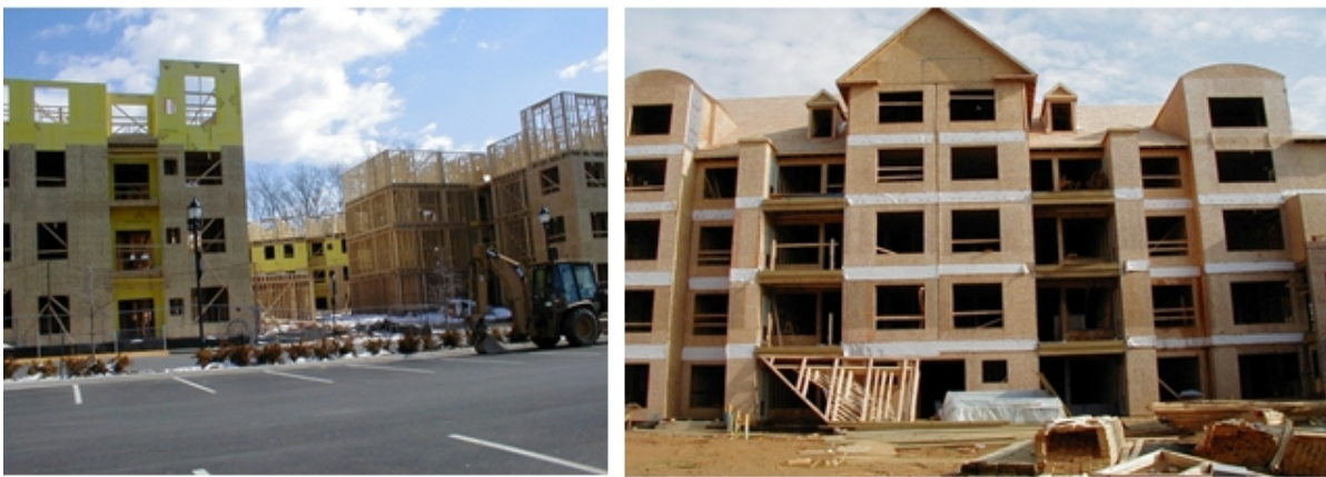
Figure 40: Residential Mid-rise Constructed Using the Platform Frame Method
