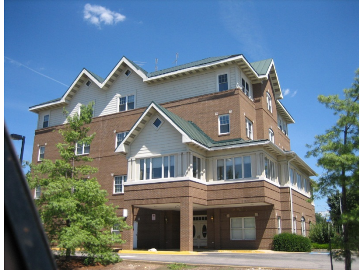
Figure 9: Lightweight Mid-rise Building Occupied as an Assisted Living Facility
