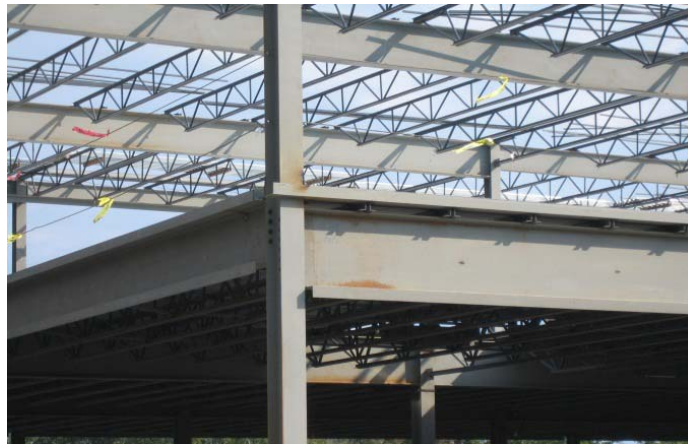
Figure 29: Non-combustible Steel-framed Building
