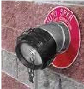
Figure 54: Large-diameter FDC
