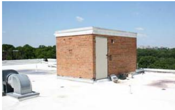
Figure 48: Roof-top Bulkhead over Stairway
