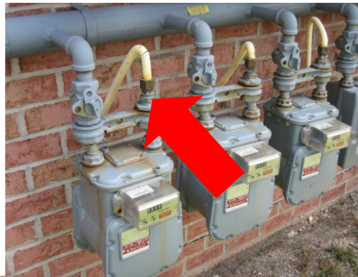
Figure 55: Flexible Light Metal Yellow Gas Pipe
