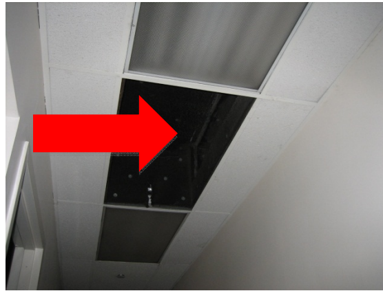
Figure 20: Hidden Pull-down Access Staircase
