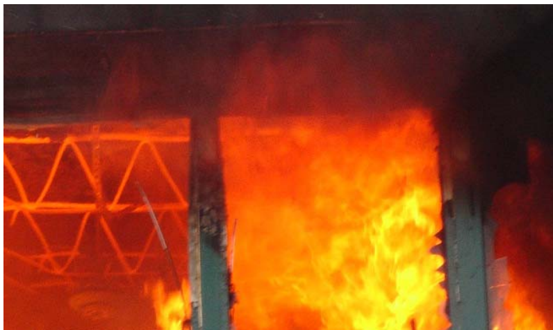
Figure 28: Truss System Losing Shape and Glowing Red Hot
