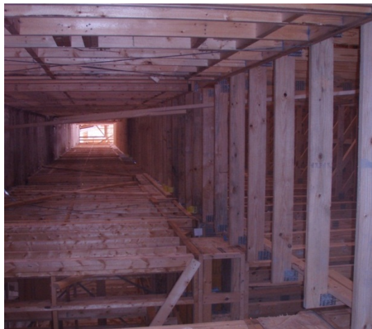
Figure 71: Cockloft Void Space
