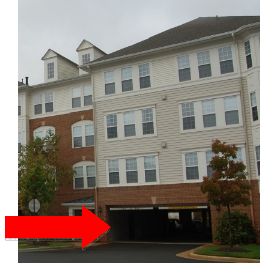
Figure 52: Parking Garage Access
