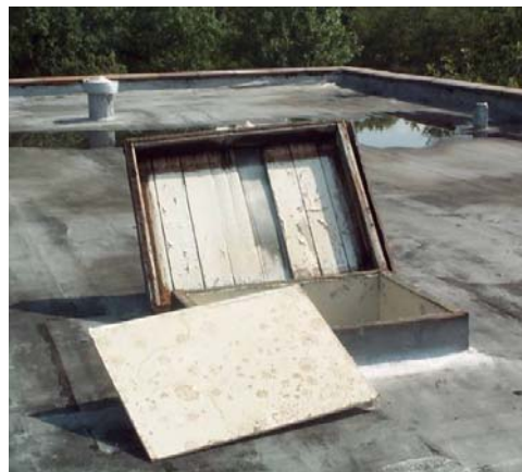
Figure 49: Roof Hatch Access to a Flat Roof
