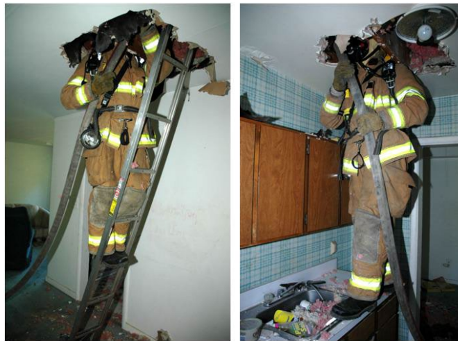
Figure 23. Gaining access to an attic fire.
