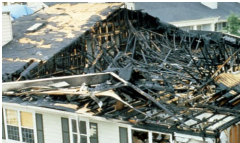
Figure 27. Dormer collapse.
