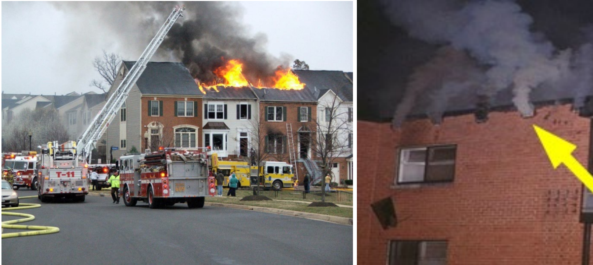
Figure 22. Example of an attic fire (left) and a cockloft fire (right) with smoke issuing from cockloft vents.
