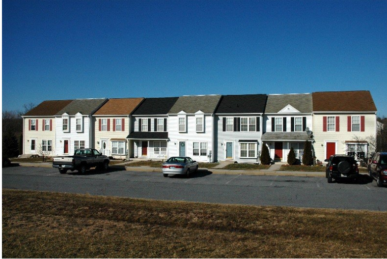
Figure 1. Typical residential townhouses.
