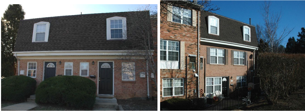
Figure 9. Over-under townhouse from side Alpha (left) and side Charlie (right).
