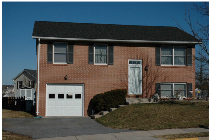
Figure 4. Typical split-foyer SFD.
