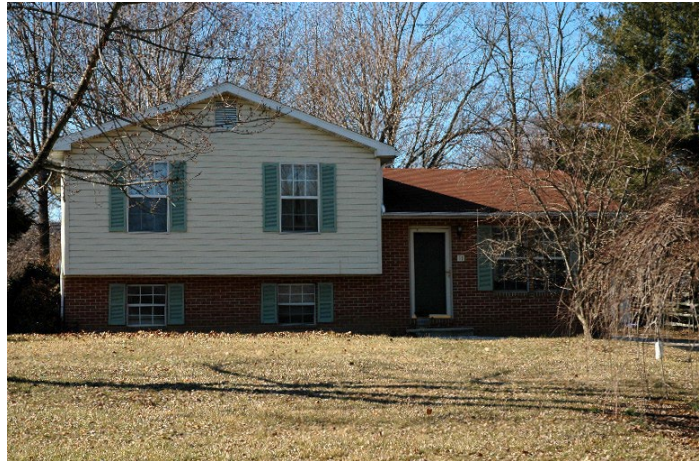
Figure 5. Typical split-level SFD.
