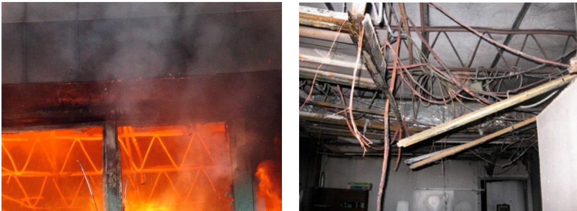
Figure 22. Steel bar joists. Beginning to fail in high temperatures (left) and frozen in place once cooled (right).
