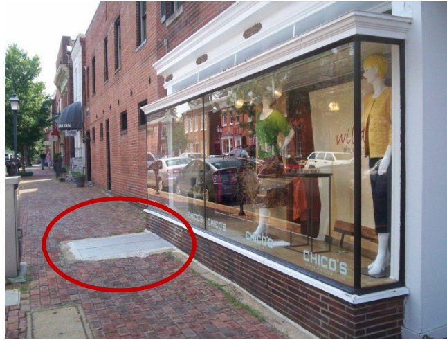
Figure 17. Basement entrance in sidewalk.
