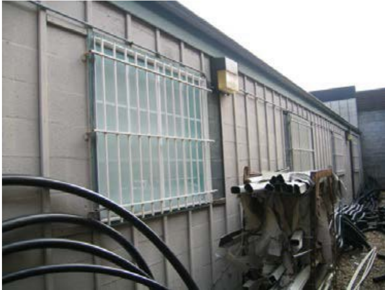
Figure 1. Rear windows secured with metal bars.
