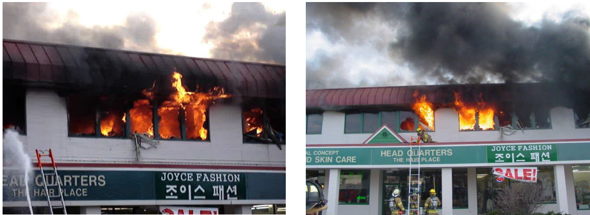
Figure 24. Fire extension via the front wall facade.
