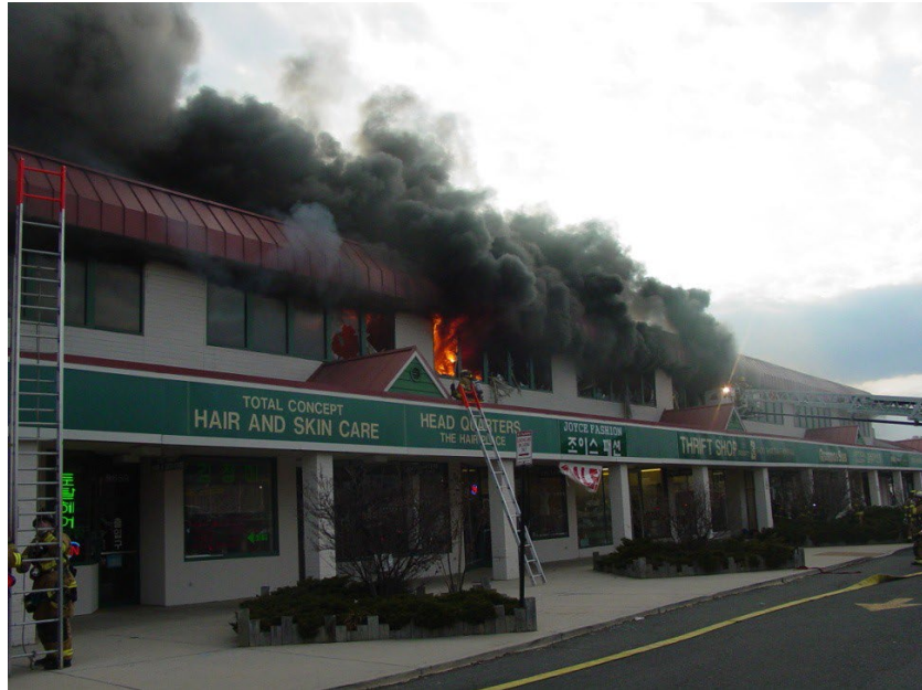
Figure 3. Horizontal fire extension in absence of firewalls.
