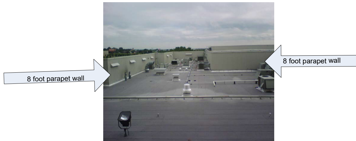
Figure 14. Parapet walls on roof edge.
