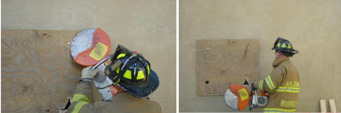
Figure 45: HUD window removal using a rotary saw.
