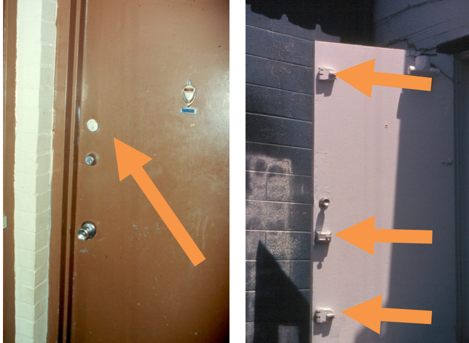
Figure 3: Outside (left) and inside (right) view of rim locks.
