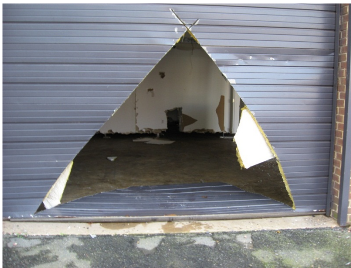
Figure 62: Inverted V cut; ensure that the cuts overlap at the top of the V.
