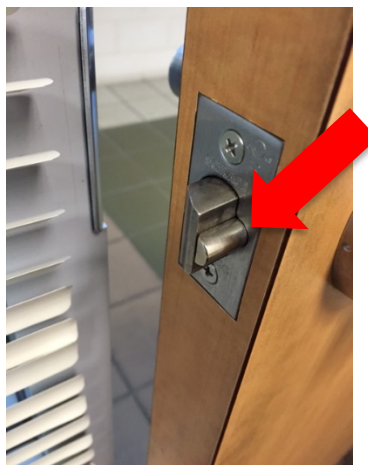
Figure 15: The dead latch contains the sliding pin alongside the latch that prevents entry without retracting the pin.
