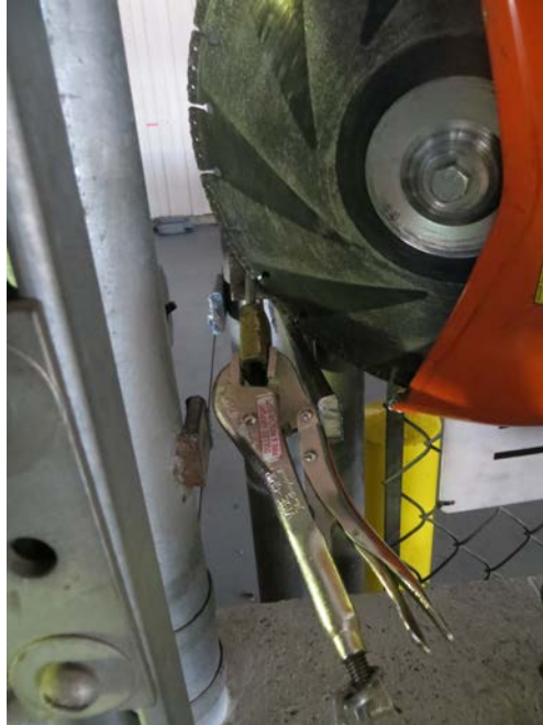
Figure 28: Use of vice grips to secure the lock prior to cutting.
