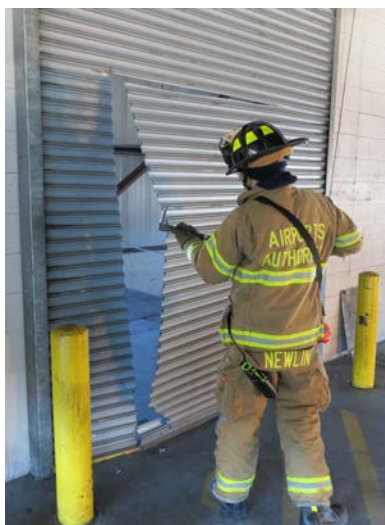
Figure 64: L cut in a roll-up door.
