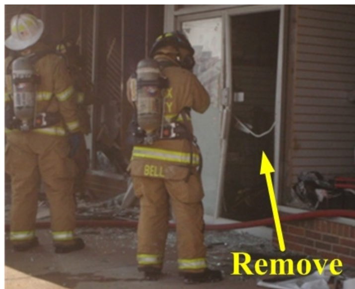
Figure 34: After removing the glass, remove panic hardware and push bars located along the door to avoid egress hazard.
