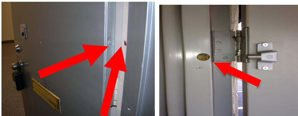
Figure 52: The multi-lock secures the door at four points in the frame. Notice the bolt from the edge of the door and corresponding keeper in the jamb.
