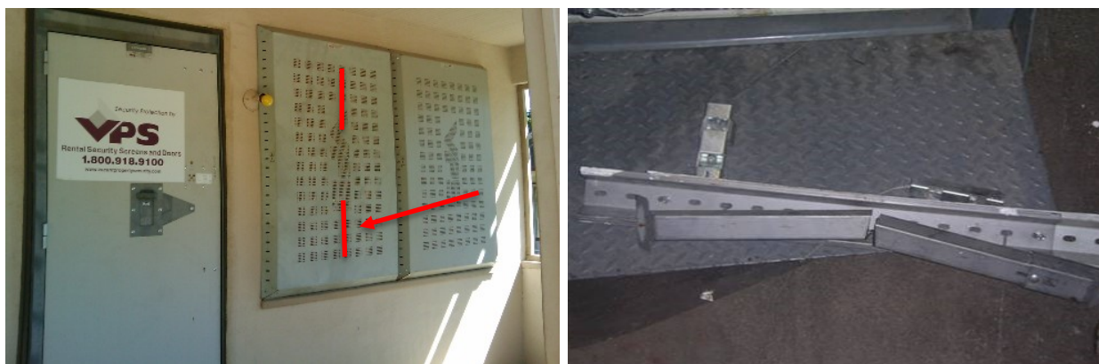
Figure 46: VPS window removal.
