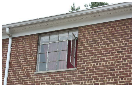
Figure 37: Casement windows shall be removed if egress is desired from the interior.
