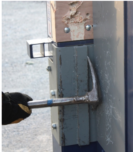
Figure 19: To gap the door, place the adz in the space between the door and jamb and apply force appropriately.
