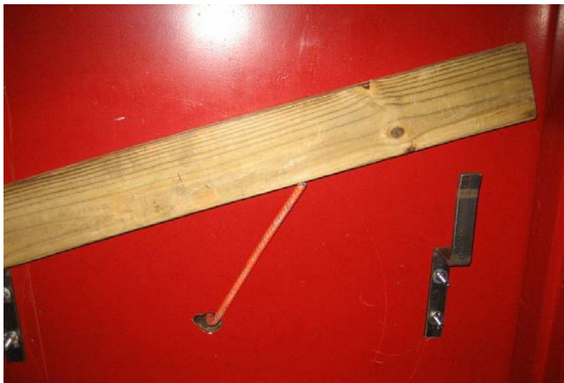
Figure 55: Rotating the rebar lifts the static drop bar out from its mounting brackets, allowing the door to open.
