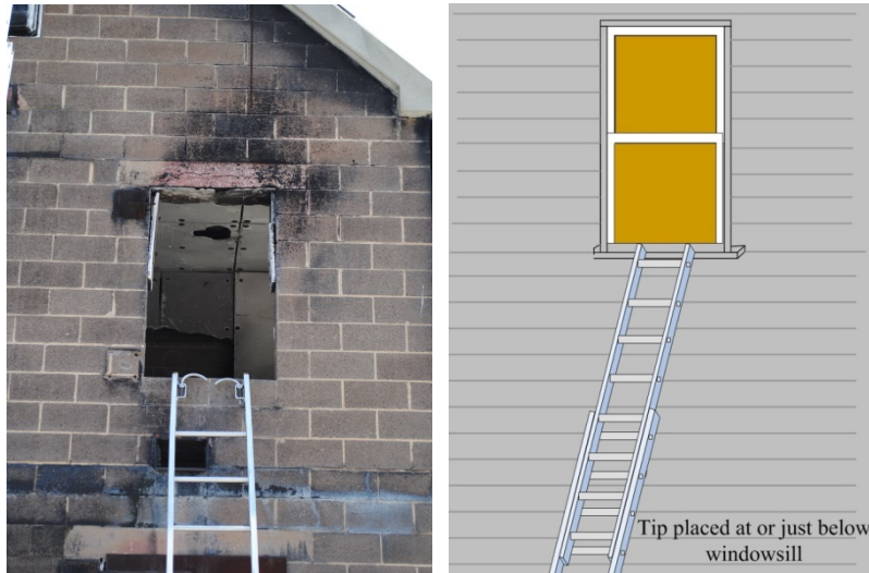
Figure 9: The preferred position for the portable ladder is at or slightly below the sill.
