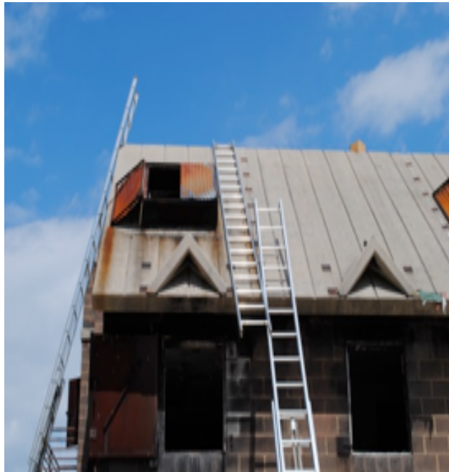
Figure 13: If operating on a peaked or pitched roof, personnel should operate off of a roof ladder placed on the roof to disperse their weight.
