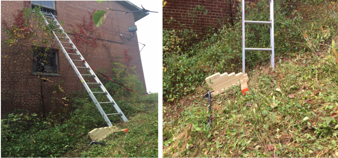
Figure 12: Use of step chock and cribbing to overcome uneven terrain for ground ladder placement.
