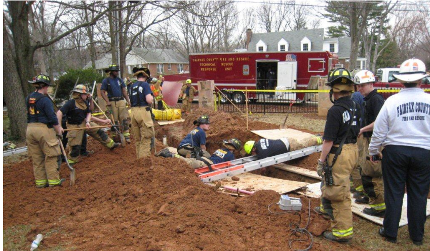
Figure 18: Using a ladder to bridge between two areas.
