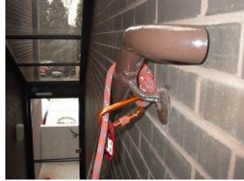
Figure 12: The fixed end of the rope should be secured to a substantial object.
