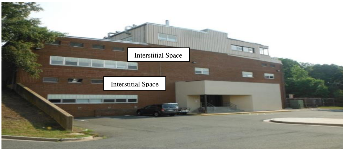
Figure 36: Another example of where interstitial space can be located in a building.
