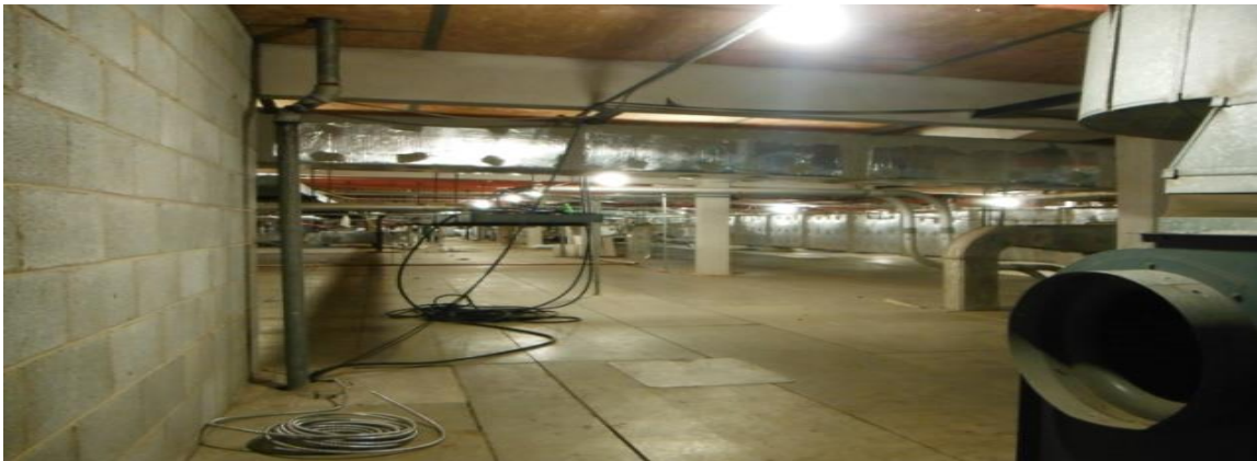
Figure 38: Example of the interior of an interstitial space.
