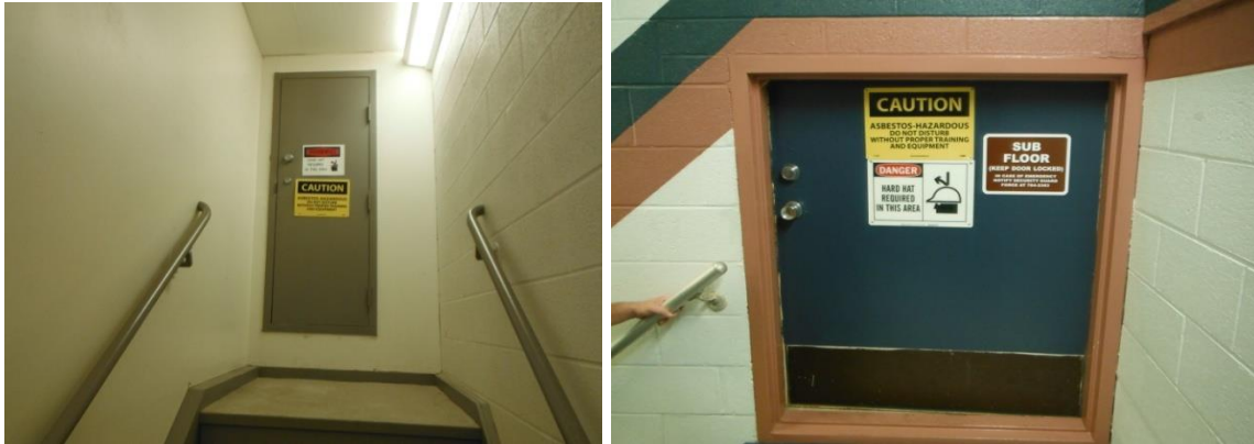
Figure 37: Examples showing that entrance doors vary in size to access the interstitial space.
