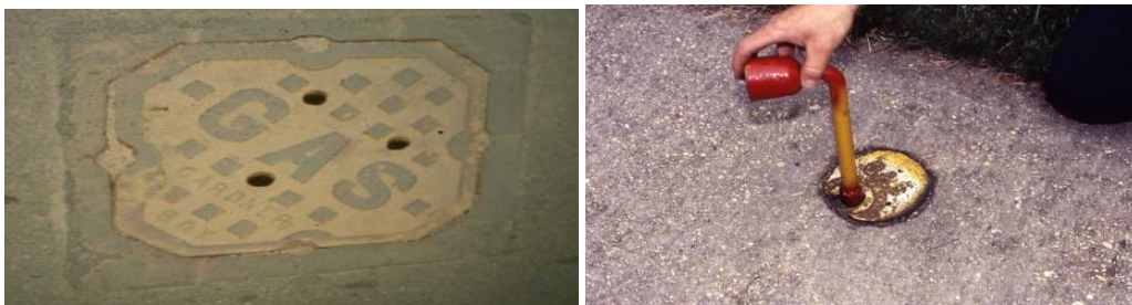
Figure 10: The image on the left shows a street valve and the image on the right shows a curb valve. Street valves should not be used.
