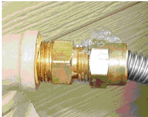
Figure 11: Locating a leak with soapy water.
