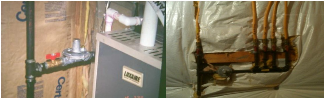
Figure 7: Examples of quarter-turn valves in residential applications.
