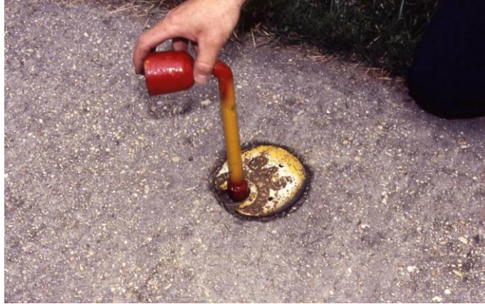
Figure 8: An example of a wrench removing a curb valve cover.
