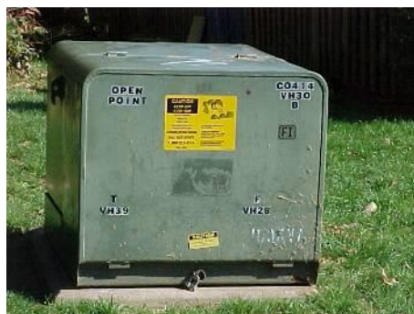
Figure 30: Ground transformer.
